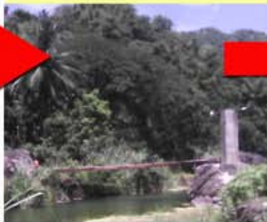
As seen from a distance: the community-made bridge that links Chesterfield to the road.
